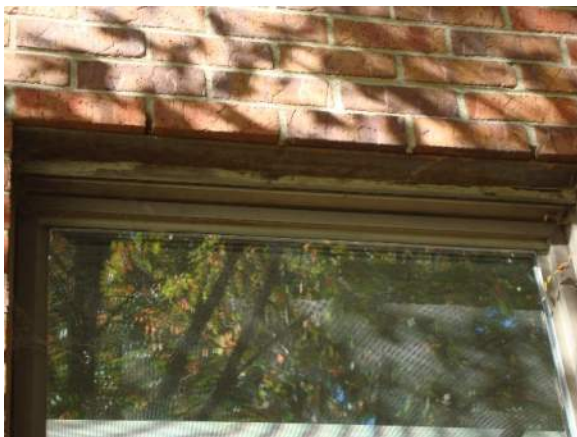
Existing Window Sealant
