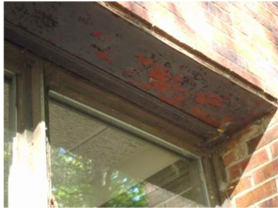
Existing Steel Window Lintel
