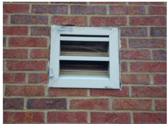
Existing Sealant at Louver
