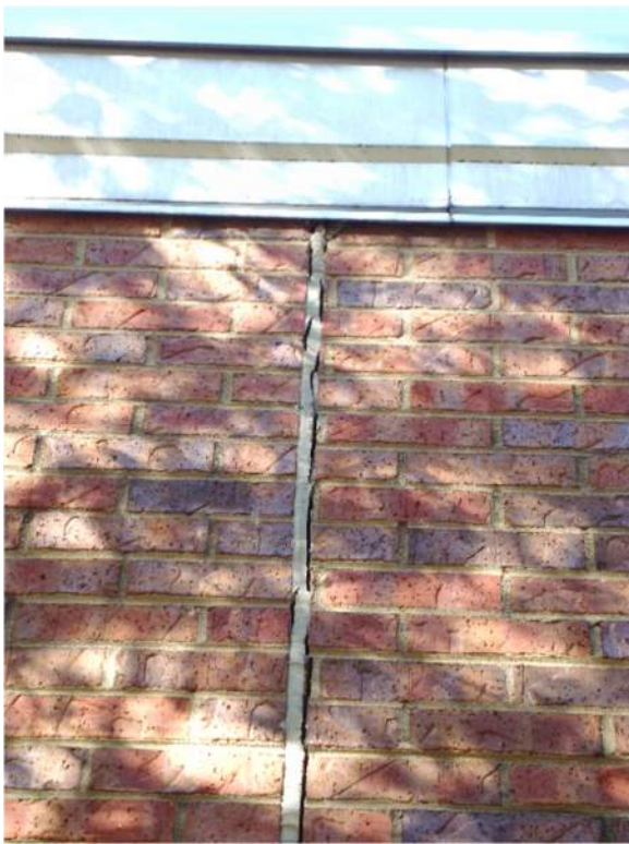
Existing Control Joint
