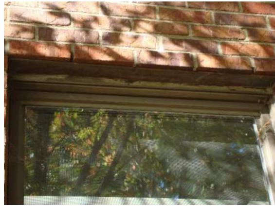
Existing Steel Window Lintel
