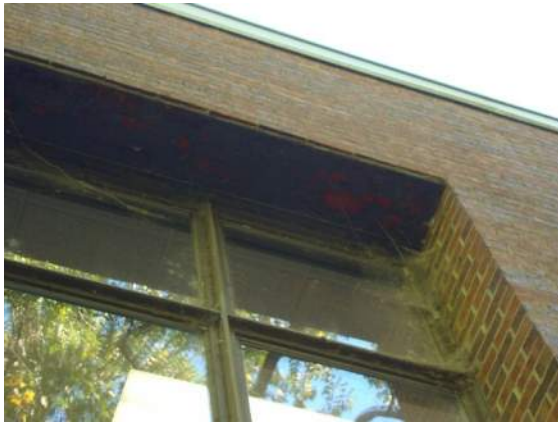
Existing Steel Window Lintel
